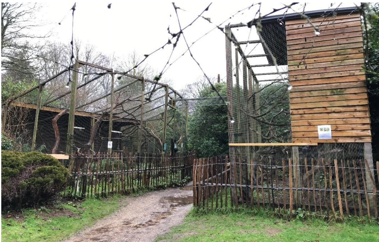
Plate 3 - New and old side with connecting run before alterations
