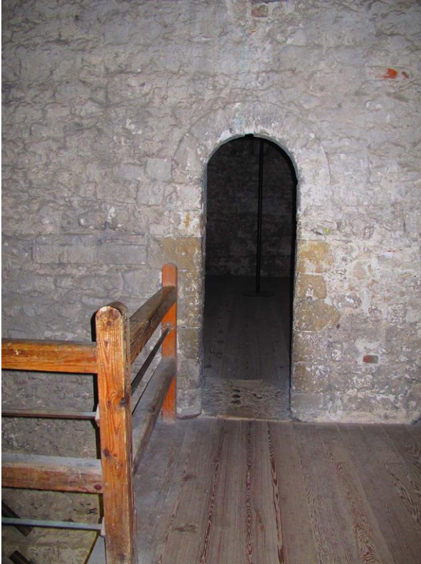
Figure 6-11: Portchester Castle, Hampshire: door in the interior spine wall, second floor of the keep, looking from the north room into the south room. Photo by the author.
